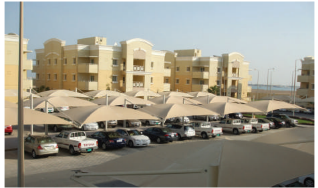
QATAR GAS - PHASE 4
